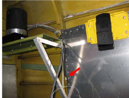
Disconnected antenna due to beacon ejection
