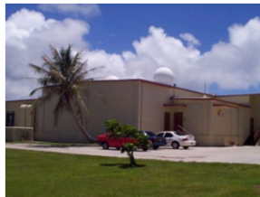
Guam Joint Region Marianas Navy Facility 2 LEO/MEOLUTs Phased Array anticipated commissioning in Spring/Summer 2024
