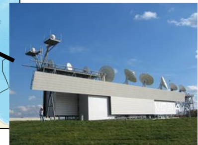
Maryland (NSOF) US Mission Control Center 2 GEOLUTs & 1 test GEOLUT 1 Test LEOLUT 1 Test LEO/MEOLUT 1 Test Phased Array under development (Rabbit Ear re- enforcement underway)
